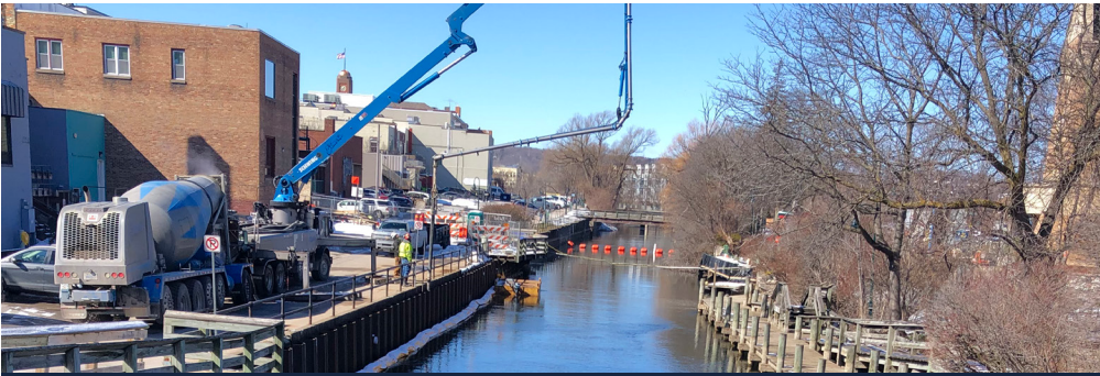
BOARDMAN RIVER SANITARY SEWER, City of Traverse City - APWA, ASCE Branch, State, and National Award Winner
